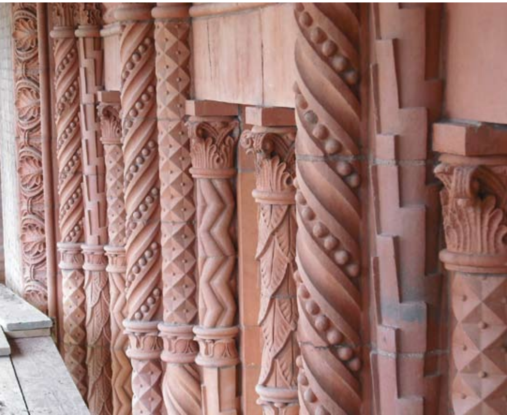
Photo: Series of terra cotta columns.
